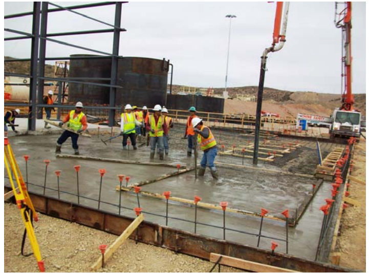
Workers Pouring Foundation of Merrill Crowe Plant in December, 2011 Source: Analyst
