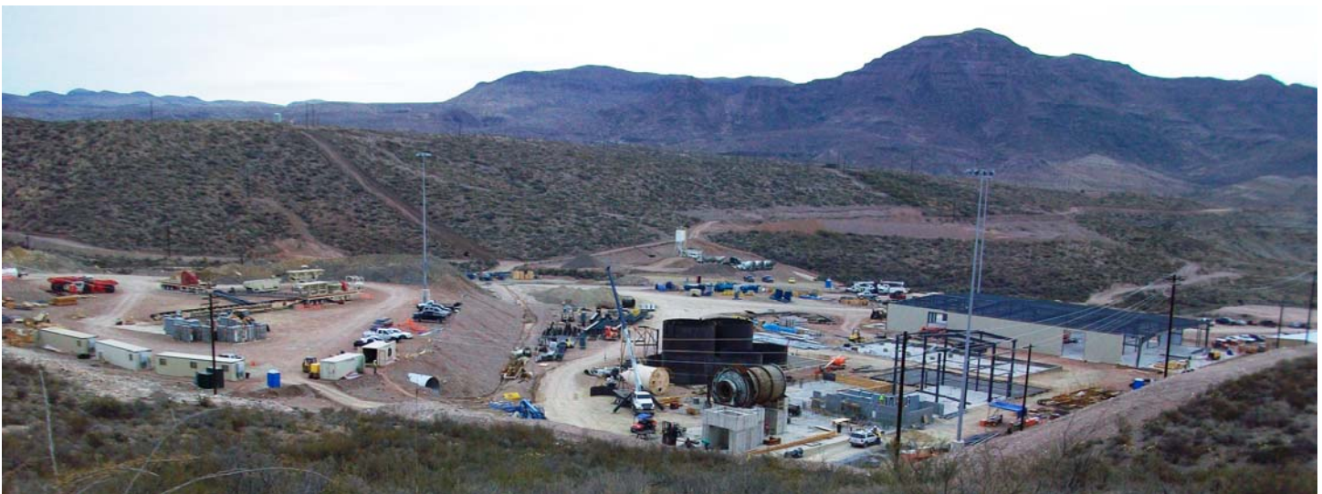
Shafter Mill Under Construction, December, 2011 (left to right) Fine Ore Pad, Mill (CIL tanks, ball mill, Merrill Crowe plant), Maintenance Shop (including warehouse, sample prep and assay lab) Source: Analyst
